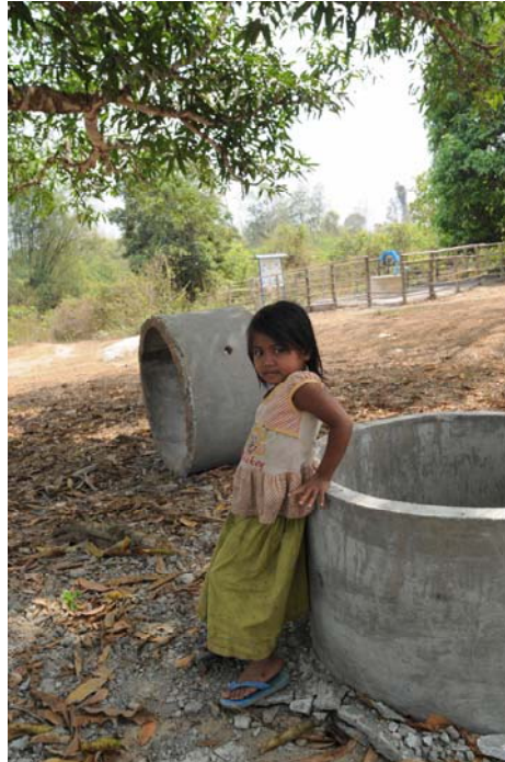
Water point construction will be followed by household latrine installations
